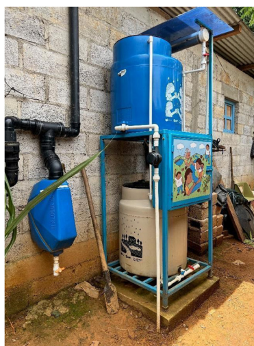
Fig. 20 The 250 L SAFEWATER system (left) with the encased LP UV lamp and activated carbon filters (right).
