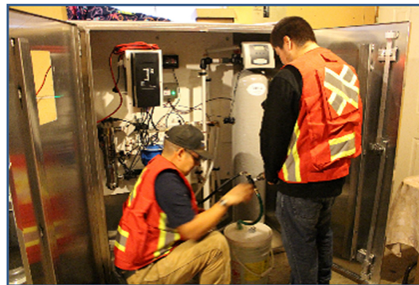
Fig. 3 The Lytton POE systems, with the low-pressure UV system, were installed in a secured enclosure, placed inside residents' homes.
