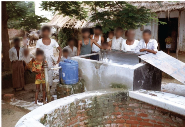
Fig. 12 View of the Bhupalpur field test. The open well in the foreground is in disuse. The hand pump to the left of the well supplies water to the blue surge tank, which feeds into a large early-design UV Waterworks unit, partly seen within the low-height concrete walls. The villager noted that the flow of this first design (60 LPM) was far larger than any hand pump flow the villager had ever encountered. This led to the more compact revised design that disinfected a water flow of 15 LPM, better matched to the UNICEF India mark-II hand pumps widely installed in the developing world.
