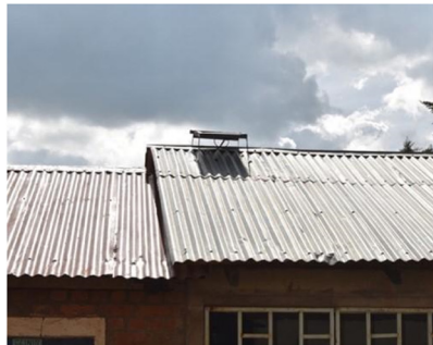
Fig. 18 System components that were designed and constructed by the welder; (left) a solar panel bracket holds the panel in place on the roof and locks so the panel cannot be stolen, and (right) a box to protect the system from tampering.
