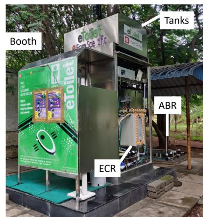
**Fig. 1** A) Schematic of the apparatus. B) Picture of the system (doors of the ECR cabinet were removed to show the ECR tank).
