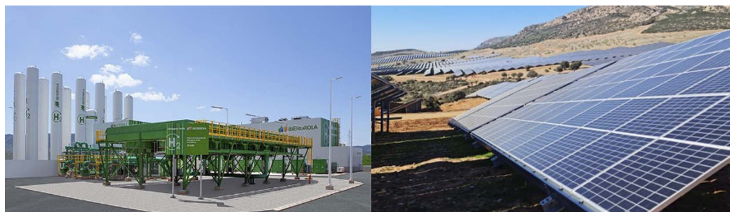
Fig. 16 Green H 2 production facility, Iberdrola, established in the year 2022 in Spain. This water electrolysis facility produces 360 kg of H 2 per hour and is powered by a solar photovoltaic plant with an installed capacity of 100 MW p. The plant also has a Li-ion battery system for streamlined and steady electrical power supply to the plant. This clearly illustrates that green H 2 production requires not only a renewable electricity generation system but also an electrical energy storage system.
