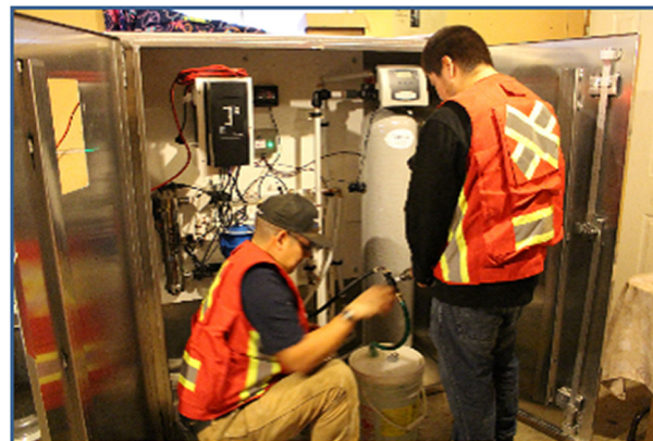
Fig. 3 The Lytton POE systems, with the low-pressure UV system, were installed in a secured enclosure, placed inside residents' homes.
