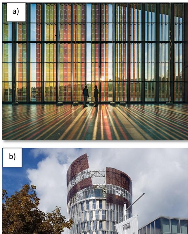
Fig. 11 (a) DSSC installation by Solaronix at center façade at EPFL campus. <https://www.epfl.ch/labs/lpi/index-html/photo-gallery-and-industrial-applications/>. (b) DSSC installations on Science Tower in Austria by H. Glass. Reproduced with permission from H.Glass S.A., copyright 2023.
