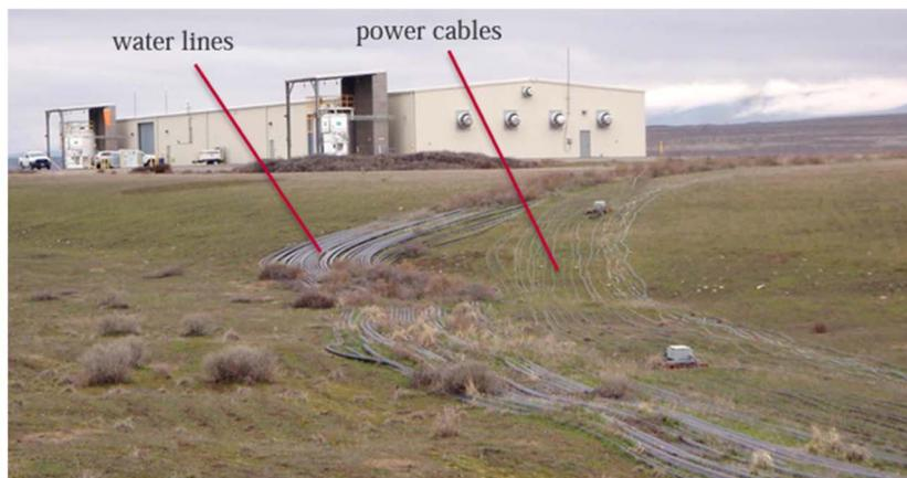
**Fig. 1** Top – Diagram illustrating the P&T process. The plume of contaminated groundwater (green) is extracted and treated, before being either pumped back into the subsurface or released as surface waters. Middle – Photo from Mackley *et al.*<sup>58</sup> showing a typical P&T extraction well at Hanford, with monitoring equipment attached. Bottom – Photo from Mackley *et al.*<sup>58</sup> showing water pipes and power cables running between a Hanford P&T facility and monitoring wells.
