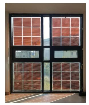
Fig. 10 DSSC BIPV mock-up. Reproduced from ref. 206. Copyright Clearance Center's RightsLink®
