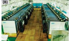
Fig. 9 Large scale CDI desalination modules produced by EST, China: (A) municipal waste water reuse desalination plant with a capacity of  $60\,000\,\mathrm{m}^3\,\mathrm{day}^{-1}$  and (B) coal mine waste water remediation plant with a capacity of  $5000\,\mathrm{m}^3\,\mathrm{day}^{-1}$ .
