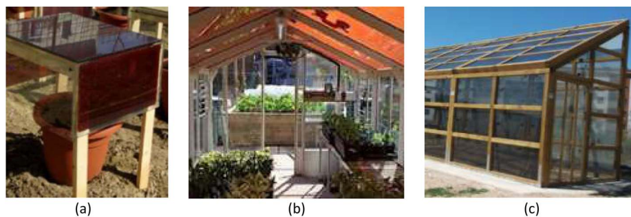
Fig. 5 a-Si APV demonstrations, (a) growth units used by Thompson et al. , 54 reproduced from ref. 54 with permission from Wiley, copyright 2020; (b) residential a-Si APV glasshouse by Polysolar, 54 reproduced from ref. 54 with permission from Wiley, copyright 2020; (c) prototype APV a-Si glasshouse used by Aira et al. , 70 reproduced from ref. 70 with permission from MDPI, copyright 2021.
