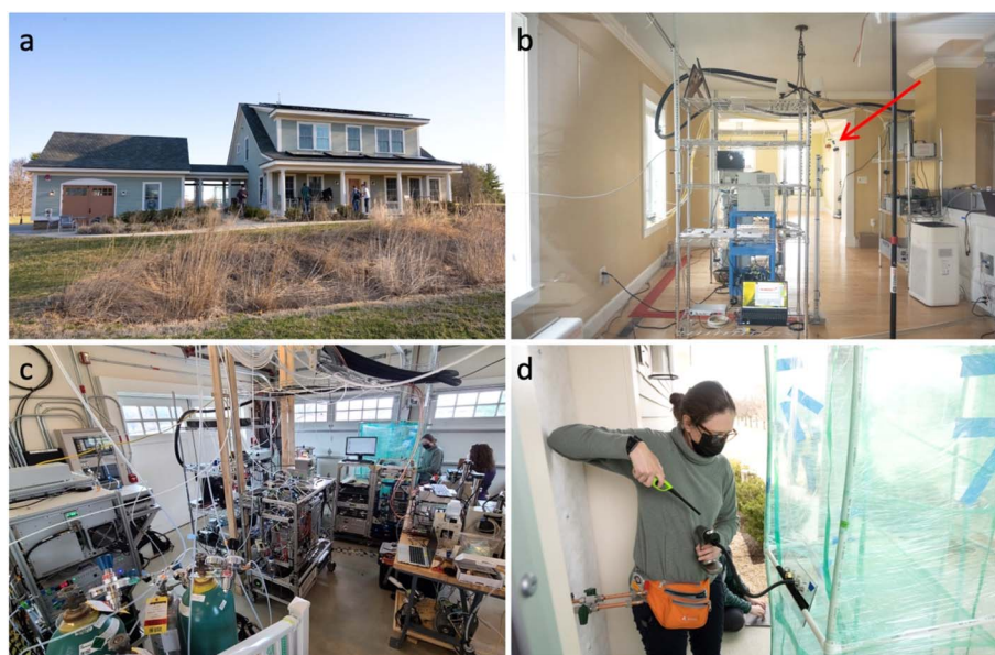
Fig. 1 Photos of (a) the NZERTF test house, with the garage holding instruments on left, joined by a breezeway to the main house. (b) The dining area contained surface samples, trace gas analyzers, low-cost sensors, and several particle sizing instruments. Inlets (marked with a red arrow) carried sample air to (c) instruments in the garage. (d) The smoke chamber in the breezeway enabled injection of aged smoke into the house. Photos (a), (b), and (d) were taken by John Eisele; (c) was taken by Dustin Poppendieck.
