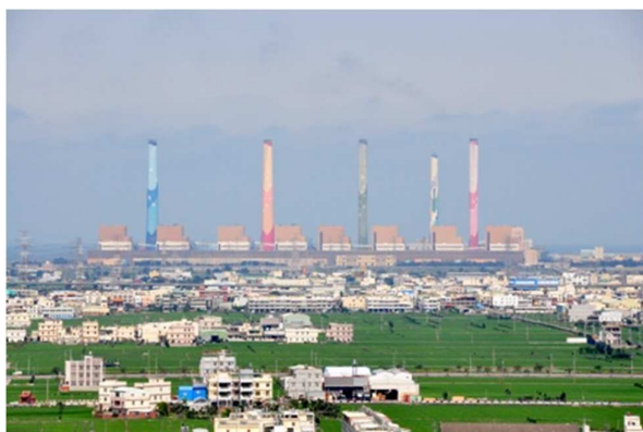
Fig. 3. Taichung Power Plant, Longjing, Taichung, Taiwan, 5,500 MW coal-fired power plant. Emissions ~40 M tonnes per annum. Stacks are 250 m high.
