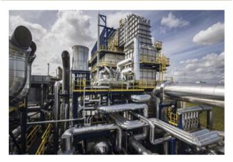
Fig. 14 One of the recent SMR-based  $H_2$  production facilities (Air Liquide's SMR-X process) in Antwerp, Belgium, produces 99.99% pure  $H_2$  at a rate of 56000 N m<sup>3</sup> per hour. The plant went into operation in April 2021. This shows the complexity of the plant and the stainless steel structures required in the form of pipes which carry hot gases.
