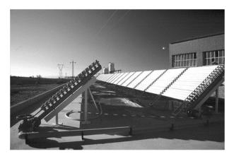
Fig. 22 One of the first pilot plants for photocatalysis, employing a slurry reactor (in a static concentrator array) installed at latitude  $40^\circ$  (Arganda del Rey, Madrid, Spain). Costing estimates in Section 1 for plant scale PCs are taken from this plant's operation. <sup>62</sup> Reproduced with permission from ref. 67. Copyright 2002 Elsevier B.V.
