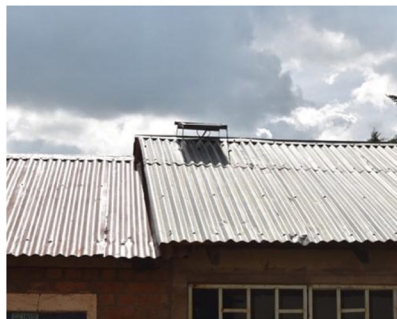
Fig. 18 System components that were designed and constructed by the welder; (left) a solar panel bracket holds the panel in place on the roof and locks so the panel cannot be stolen, and (right) a box to protect the system from tampering.
