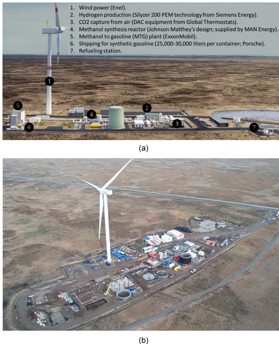
Fig. 22 (a) Schematic of the Haru Oni project, southern Chile, which will produce industrial-scale e-methanol starting from the end of 2022. Adapted from ref. 75. (b) Actual site of the Haru Oni project. From ref. 109.
