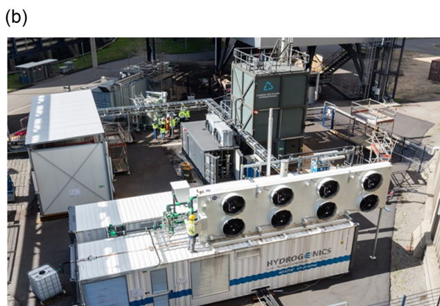
Fig. 19 (a) Schematic of the MefCO 2 plant 77 and (b) the actual pilot-scale MefCO 2 plant (right) at RWE's lignite-fired coal power plant in Niederaussem, Germany. 104
