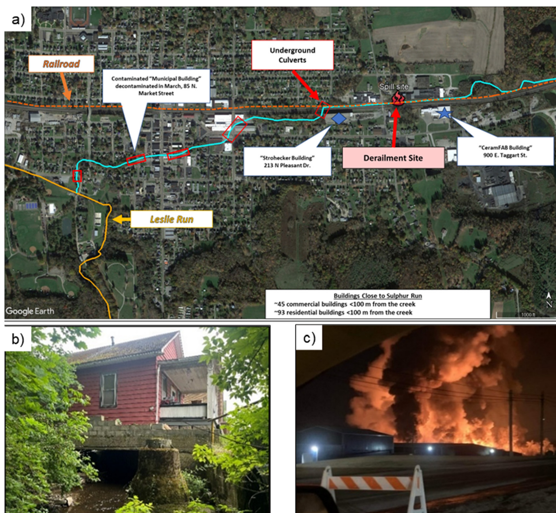
Fig. 1 a) Map showing the derailment site, culverts, and contaminated buildings near Sulphur Run, b) chemicals released from the derailment entered Sulphur Run and flowed into concrete culverts underneath residential, commercial, and municipal buildings, c) image of the chemical fire visible from East Taggart Street by the CeramFAB Building on February 3, 2023. This image was taken before the open burn was conducted February 6, 2023.
