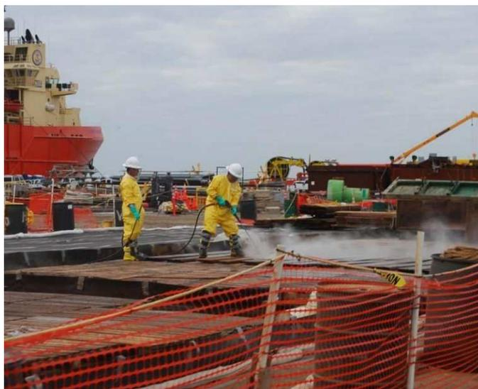
**Figure 5.** Workers in Louisiana using limonene-based cleaning agent PES-51 to decontaminate equipment used to clean large vessels following the Macondo well blowout and Deepwater Horizon explosion on April 20, 2011. [Image reproduced from Ref.20, with kind permission].
