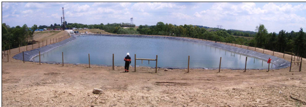
Figure 4: Hill top pit incised into subgrade with geomembrane liner
