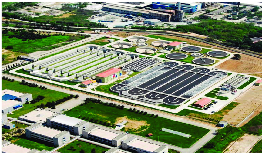
Fig. 1 Municipal WWTP facility located in Gebze-Kocaeli, Türkiye.
