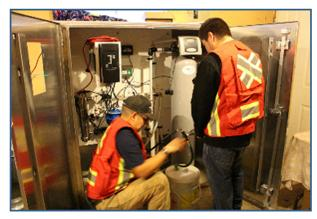
Fig. 3 The Lytton POE systems, with the low-pressure UV system, were installed in a secured enclosure, placed inside residents' homes.
