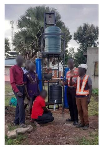
Fig. 32 ASEI and AquiSense Technologies water treatment and delivery system.
