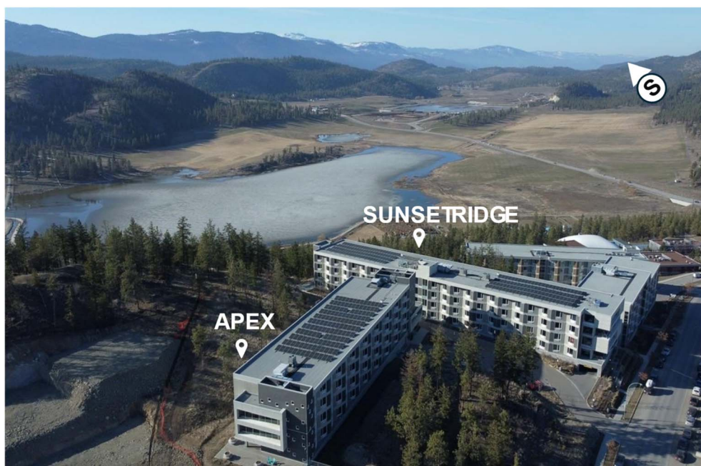
Fig. 2 Rooftop layout and surrounding area of the VEDA exclusive student living residences. 40
