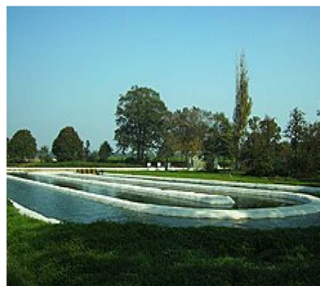
Fig. 3 Open race way pond.
