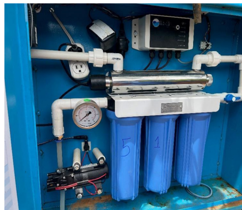
Fig. 20 The 250 L SAFEWATER system (left) with the encased LP UV lamp and activated carbon filters (right).
