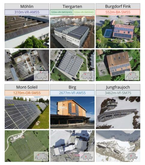
Fig. 2 System photos, showing the profile view (top) and aerial view (bottom). Approximate location in Switzerland is indicated in the bottom right corner. The Tiergarten system is separated in the East and West parts of the rooftop in the data and results. Site IDs are indicated below the system name, following the defined format: [Altitude]–[Mounting Config.]–[Module Type], see Table 1.
