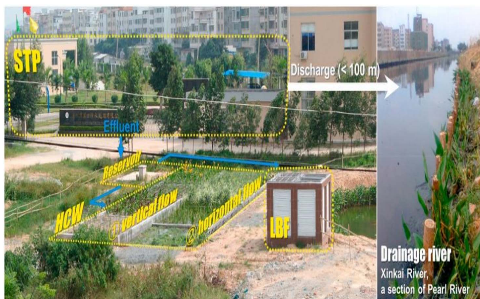
Fig. 21 Layout of the full-scale system for purifying STP discharge (Copyright Elsevier 2021) ref. 190.
