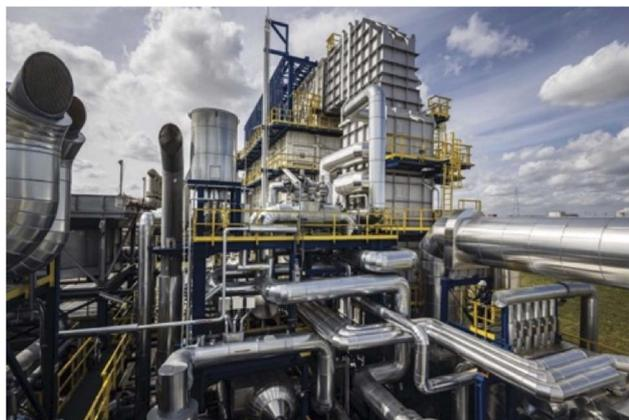
Fig. 14 One of the recent SMR-based H<sub>2</sub> production facilities (Air Liquide's SMR-X process) in Antwerp, Belgium, produces 99.99% pure H<sub>2</sub> at a rate of 56000 N m<sup>3</sup> per hour. The plant went into operation in April 2021. This shows the complexity of the plant and the stainless steel structures required in the form of pipes which carry hot gases.
