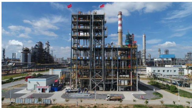
Fig. 20 Photo of the industrial pilot plant to produce short olefins via the OX-ZEO to olefins (OXZEO ® -TO) process, located in Shaanxi, China. 489
