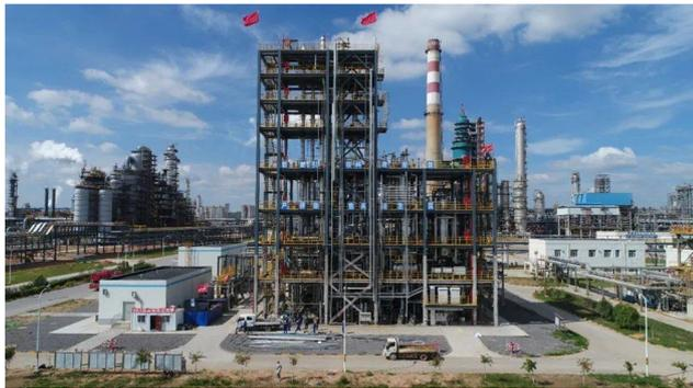
Fig. 20 Photo of the industrial pilot plant to produce short olefins via the OX-ZEO to olefins (OXZEO<sup>®</sup>-TO) process, located in Shaanxi, China.<sup>489</sup>
