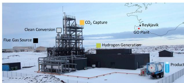
Fig. 18 CRI's GO plant in Svartsengi, Iceland, which uses CO<sub>2</sub> captured from the nearby geothermal power plant (in background) and H<sub>2</sub> produced through electrolysis to form renewable methanol. From ref. 103.
