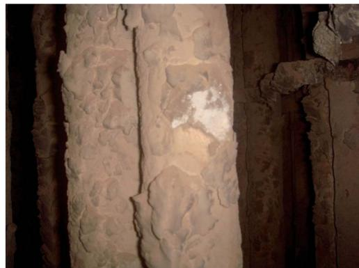
Fig. 2 Deposits on high temperature superheater.
