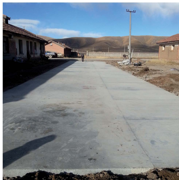
Fig. 17 Field test section.
