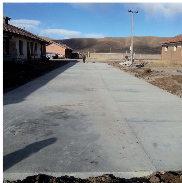
Fig. 17 Field test section.
