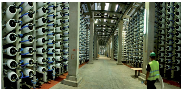
Fig. 1 Hadera RO Desalination Plant, Israel, 127 million \text{m}^3 year ^{-1} . The Hadera seawater desalination plant in Israel, among the worlds most efficient, contains tens of thousands of RO membrane cartridges. Courtesy of IDE Technologies Ltd.
