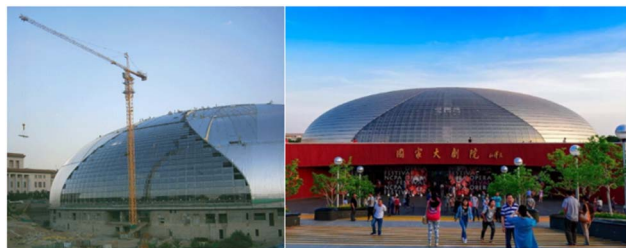
Fig. 5 Self-cleaning dome glass of China National Opera House under construction and appearance drawing. 82
