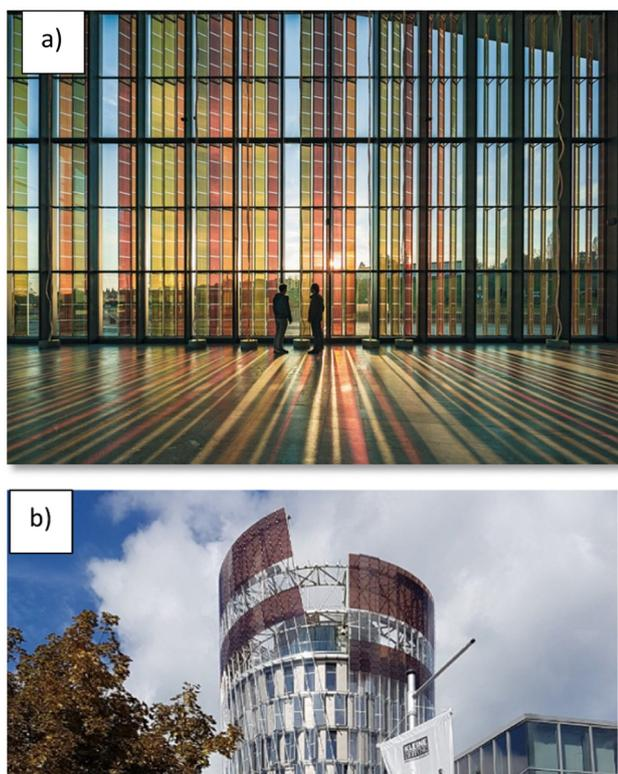
Fig. 11 (a) DSSC installation by Solaronix at center façade at EPFL campus. <https://www.epfl.ch/labs/lpi/index-html/photo-gallery-and-industrial-applications/>. (b) DSSC installations on Science Tower in Austria by H. Glass. Reproduced with permission from H.Glass S.A., copyright 2023.
