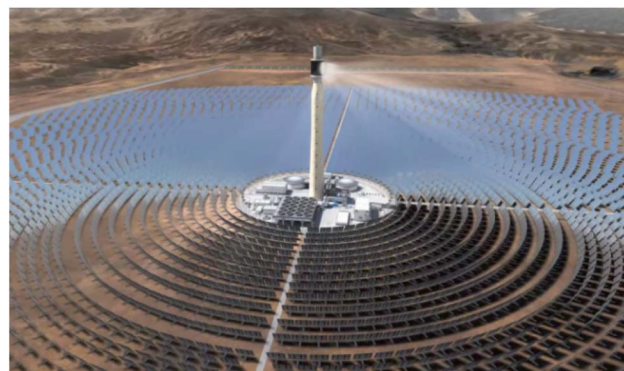
Fig. 6 Aerial view of the Ouarzazate Solar Power Station in Morocco. Image adapted from cited ref. 76.
