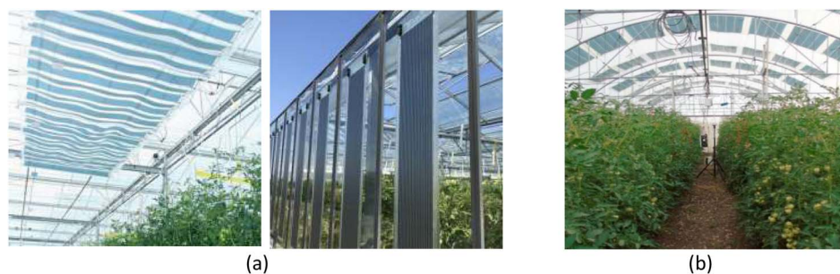
Fig. 6 Flexible OPV modules demonstrated in greenhouses (a) ASCA® modules deployed in an industrial greenhouse, France, reproduced from ref. 77 with permission from ASCA, copyright 2021; (b) testing of OPV modules installed on a polytunnel roof, reproduced from ref. 78 with permission from Elsevier, copyright 2022.
