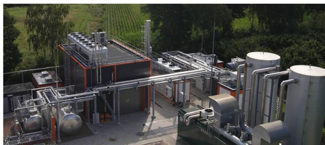
Fig. 24 Actual site of the 350 tpa of SAF production plant at Werlte in Germany, including the electrolysis system that forms the core of the plant.<sup>114,115</sup>
