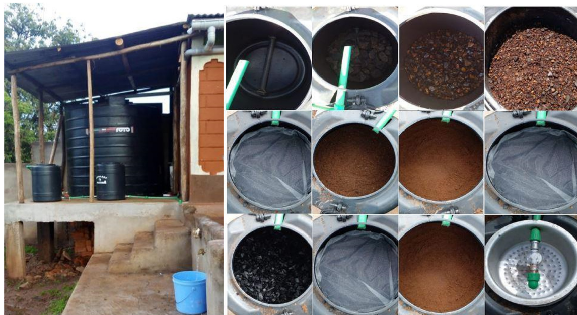
Fig. 17 (Left) Rainwater collection, filtration and disinfection system. (Right) Biosand and biochar layers within the filtration system.
