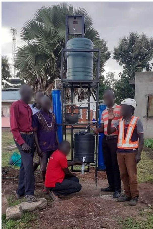
Fig. 32 ASEI and Aquisense Technologies water treatment and delivery system.
