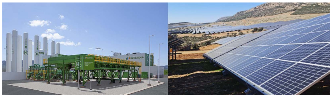
Fig. 16 Green H 2 production facility, Iberdrola, established in the year 2022 in Spain. This water electrolysis facility produces 360 kg of H 2 per hour and is powered by a solar photovoltaic plant with an installed capacity of 100 MW p. The plant also has a Li-ion battery system for streamlined and steady electrical power supply to the plant. This clearly illustrates that green H 2 production requires not only a renewable electricity generation system but also an electrical energy storage system.
