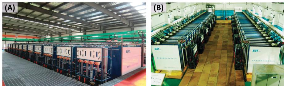
Fig. 9 Large scale CDI desalination modules produced by EST, China: (A) municipal waste water reuse desalination plant with a capacity of 60 000 m<sup>3</sup> day<sup>-1</sup> and (B) coal mine waste water remediation plant with a capacity of 5000 m<sup>3</sup> day<sup>-1</sup>.
