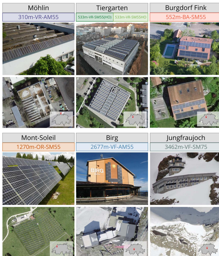
Fig. 2 System photos, showing the profile view (top) and aerial view (bottom). Approximate location in Switzerland is indicated in the bottom right corner. The Tiergarten system is separated in the East and West parts of the rooftop in the data and results. Site IDs are indicated below the system name, following the defined format: [Altitude]-[Mounting Config.]-[Module Type], see Table 1.
