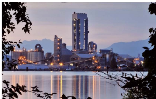
Cement -Lafarge Canada Inc. (Richmond) t CO 2 e = 658,346 in 2018 report Table 2
