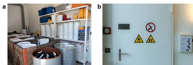
Fig. 4 Ventilated central storage for special waste, including nanowaste. a: Collection area for full nanowaste containers prior to pick-up by a treatment company. b: Example of a storage room built to comply with ATEX regulations (explosive atmospheres). Note the secure design (watertight floor, restricted access, device drop-off box for ignition sources).
