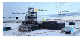
Fig. 18 CRI's GO plant in Svartsengi, Iceland, which uses  $\rm CO_2$  captured from the nearby geothermal power plant (in background) and  $\rm H_2$  produced through electrolysis to form renewable methanol. From ref. 103.
