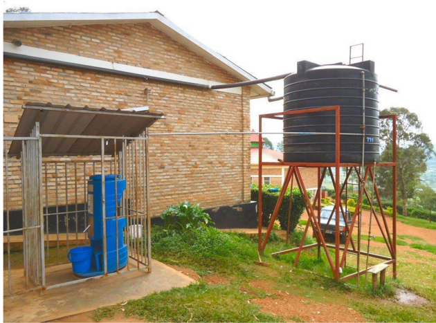
Fig. 25 A Naiade (on the left) and rainwater harvesting tank on a primary school in Kigali, serving 240 children and 20 staff members.
