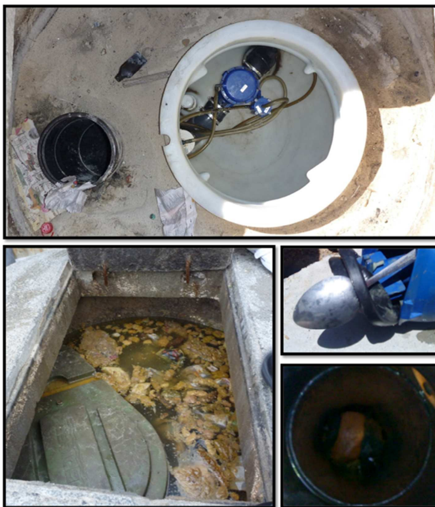
Figure 1: Clockwise from the top: (a) A collection chamber in Kosovo's vacuum system, with the sump on the left and the sensor unit on the right (Taing, 15 April 2011); (b) a damaged interface valve diaphragm (Cornelius, 26 June 2009); (c) a brick in the sump (Cornelius, 28 February 2010); and (d) a flooded chamber (Taing, 7 June 2010).
