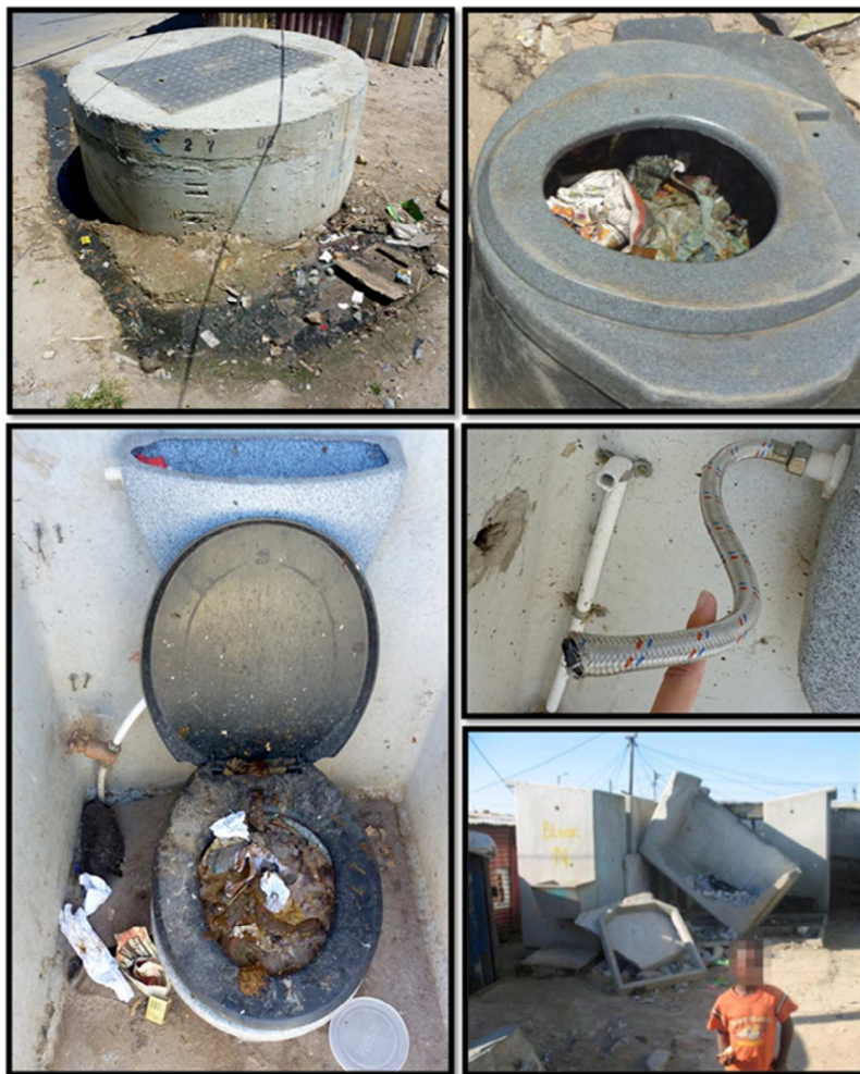
Figure 2: Clockwise from top: (a) sewage seeping from a collection chamber (Taing, 29 November 2010). While (b) container toilets are unsightly and smell, Kosovo residents preferred them to the ineffective vacuum toilets because the contents of the plastic containers did not seep into the surrounding environment. Residents, who were dissatisfied with the malfunctioning system, also (c) cut water supplies of units to deter usage (Taing, 11 November 2010) and (d) destroyed toilets in protest (Pan, 30 May 2010). But, as (e) the photo of a full but disconnected toilet indicates, some nevertheless continued to use the vacuum toilets (Taing, 15 April 2011).
